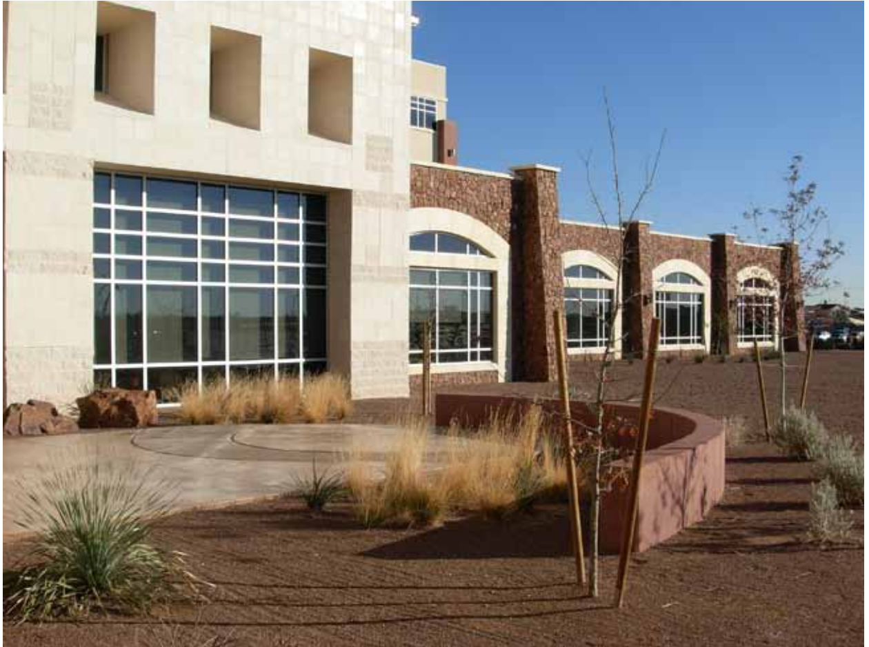
In winter, the cast-in-place concrete seat wall and paving provide a sunny sitting area, extending the interior lobby forms outward. As this matures, deciduous Texas Red Oak will allow in some sun, while dormant Blue Grama clumps highlight the Sotol. A future water feature will create cool sounds in summer, when all is in leaf or flowering.
